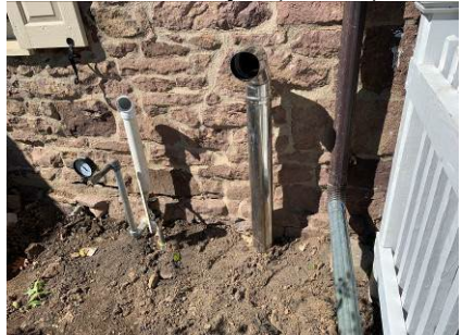
New Gas Pipes (outside)
