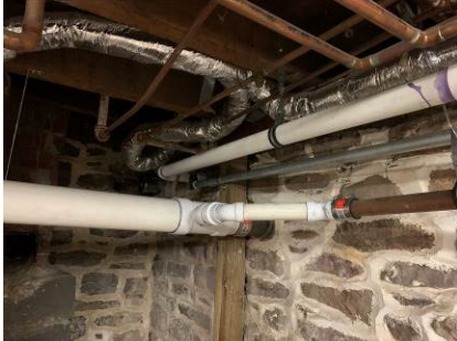
New Gas Pipes (inside)
