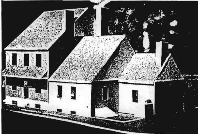
Figure 3. 1810 period showing newly constructed one story stone South Portion and new kitchen with bake oven.
