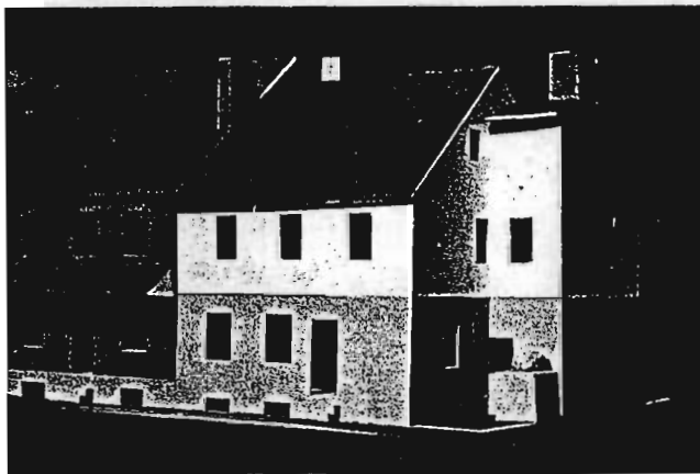
Figure 4. Model of the Court Inn c1840. At this time the building was essentially the same size as exists today.
