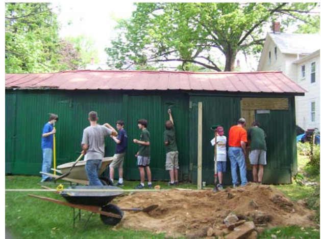
Scouts of Troop #380 hard at work repainting the barn.
