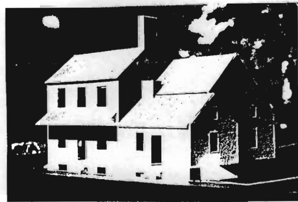
Figure 5. Period D, c. 1745. A frame shed roof addition has been attached to the east face of Period A.
