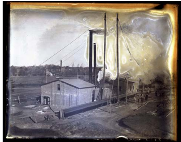
A view of the Newtown Electric Light & Power Company from the third floor of the Worstall Mill. Note the 60 foot smoke stack ready to be raised into position and the Stocking Works which is visible in the background.
