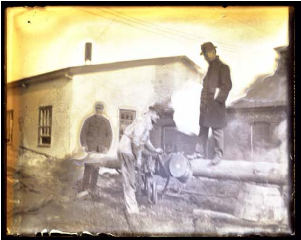
Workers readying the pole, pulley and cable system used to raise the 60 foot smoke stack into position.
