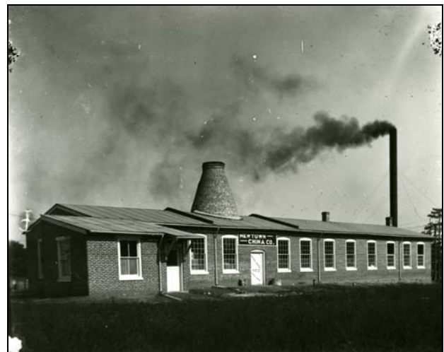
A view of the Newtown China Company located at 451 South State Street. Note the 60-foot smoke stack to the Newtown Electric Light and Power Company in the background, further evidence of its position in Newtown.
